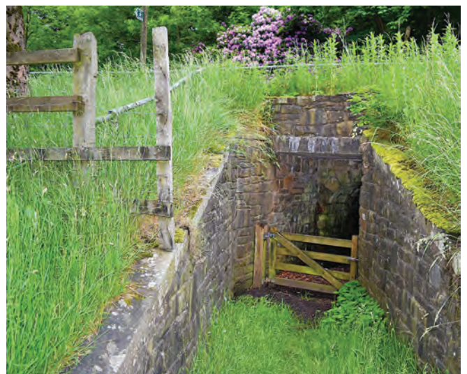
Southwest approach to the subway
